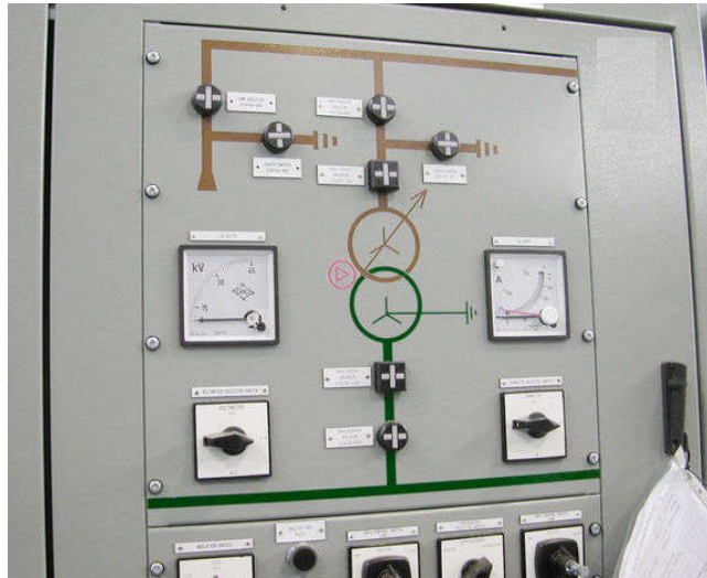
Industrial Vinyl Mimic Panel with Ammeter & Voltmeter Selector Switches Vinyl's in colours Brown & Green.
