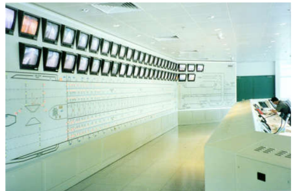
Fig. H shows the combination larger mosaic mimic panels linked to, monitored and controlled by operators from control desks.
