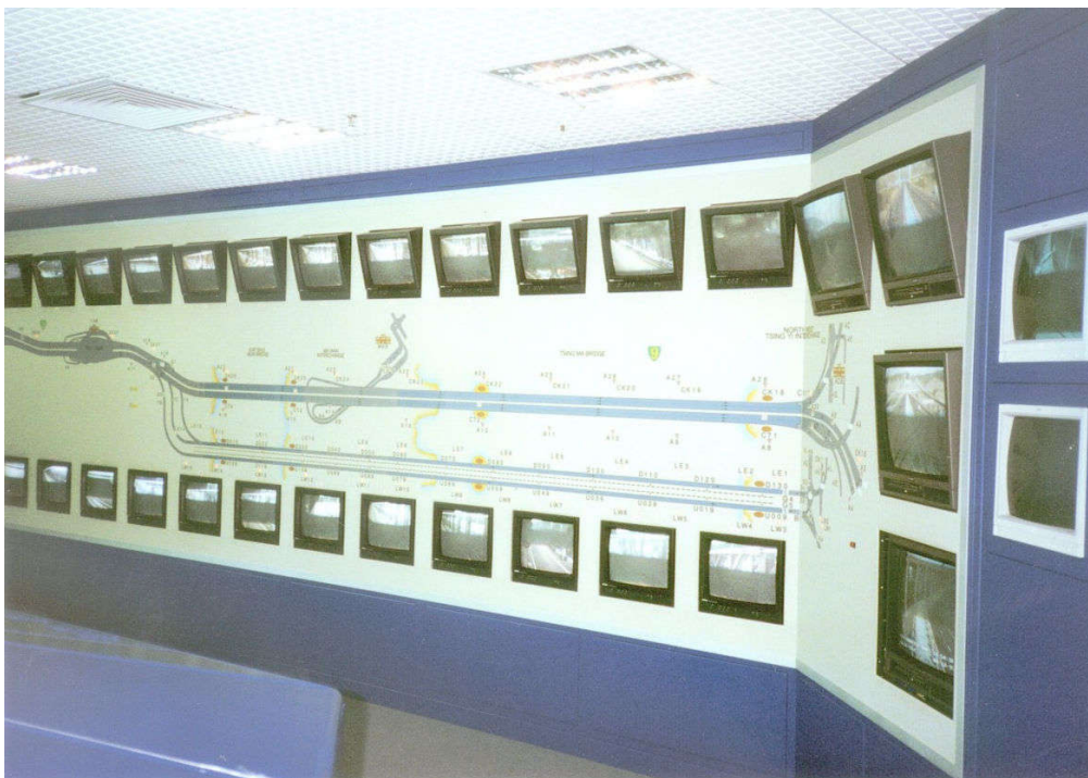
Mosaic mimic panel of the route to the Hong Kong Airport Project 1996-1997.
