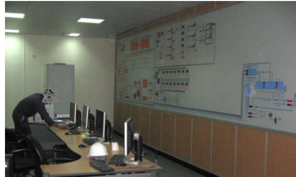
Fig. G shows the convenience of operating larger mosaic mimic panels with operator control desk & monitors.
