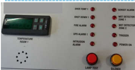
Engraved temperature with alarm system fitted with LEDs for a mimic panel
