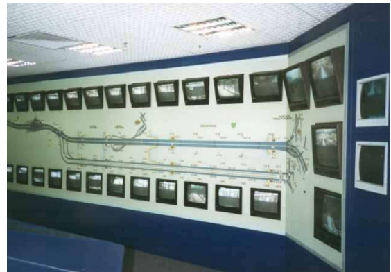
Fig. A shows the convenience of fitting monitors directly into our mosaic (Hong Kong airport bridge)
