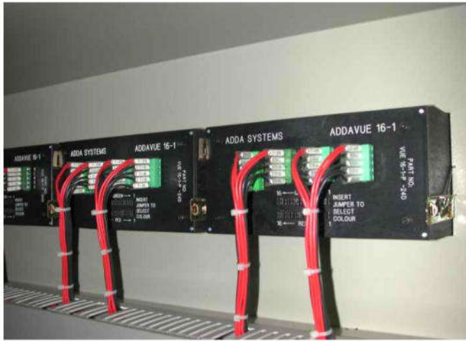
Rear view of ADDAVUE 16-way display units
