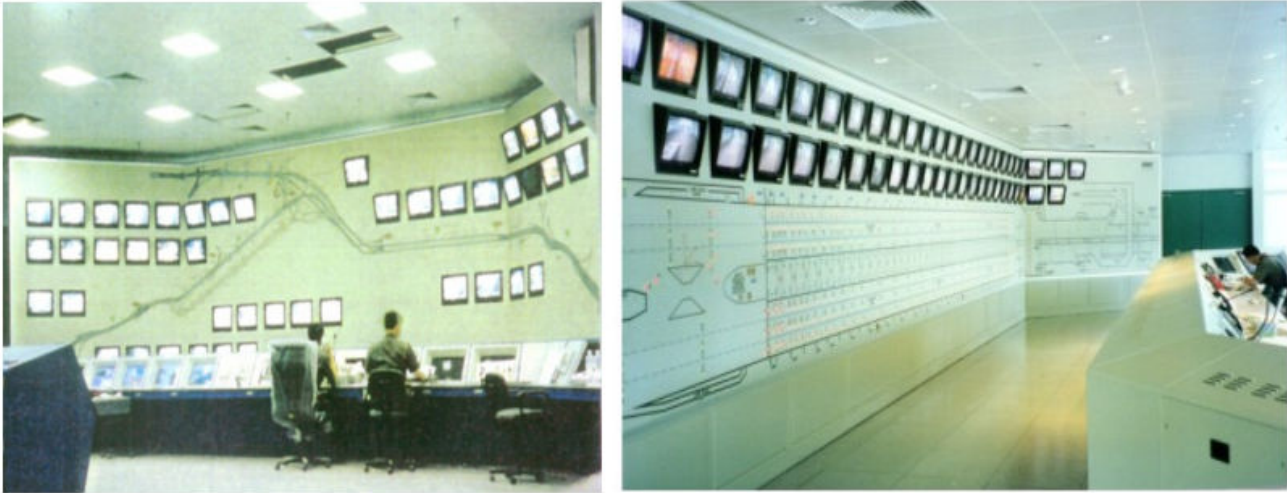
Project: Hong Kong massive wall-to-wall Mosaic Mimic Panel combined with Panel facing Control Desk
