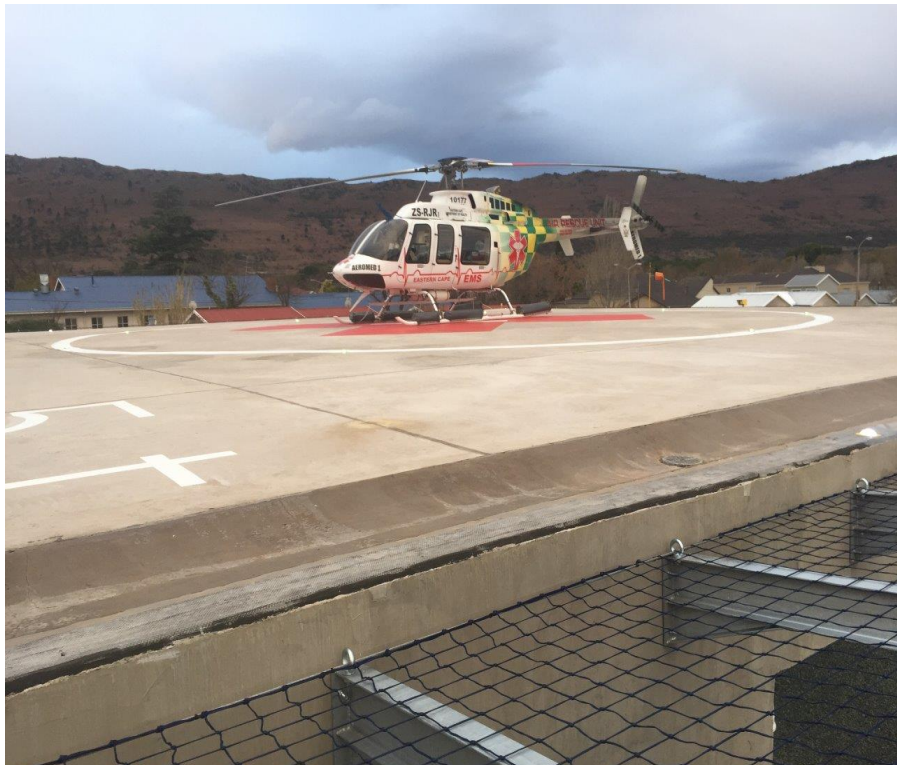
Roof-top Helipad with Safety Net
