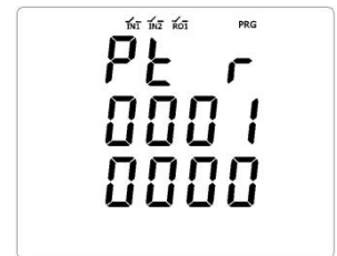
Potential Transformer Ratio
